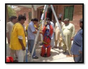
manhole. Sewer man smoothly enters and gets out with the help of this system from the manhole by maintaining a balance. It is very easy to operate the winch with small force. The sewer man does not lose his balance and can easily be withdrawn from the manhole. Practical demonstration was given to the trainees at site.
