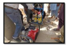
requirements. Each cylinder can work for 2 hours and if pressure is reduced to a certain level, beep is heard by the sewer men &the staff standing outside the manhole should immediately withdraw the worker from the manhole.
