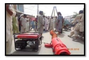
again. If the harmful gases have been removed and ample amount of oxygen is present in the manhole then the supervisor should allow the sewer men to enter the manholes.
